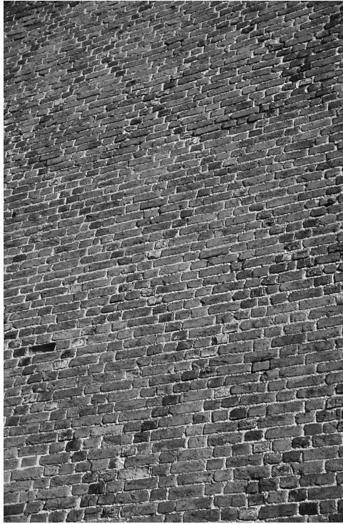
Figure 11.9 Świecie, Northern Poland, Castle façade, Pattern of the black-fired bricks (Tomasz Torbus 1996)
